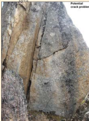
Potential Crack Problem
